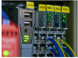
State-of-the art SPS control
